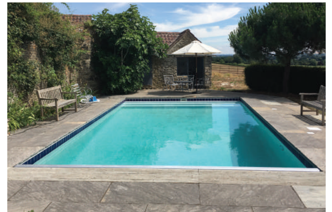
2670 | PRIVATE CLIENT, BATH PROJECT | POOL RENOVATION
