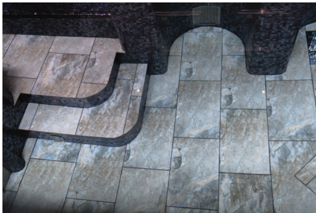
2697 | PRIVATE CLIENT, CHELTENHAM PROJECT | POOL & HOME SPA
