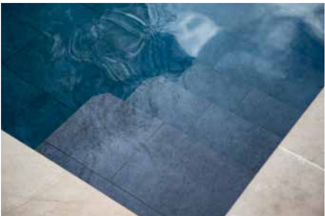
2838 | PRIVATE CLIENT, BRISTOL PROJECT | OUTDOOR TILED POOL & TILED SPA
