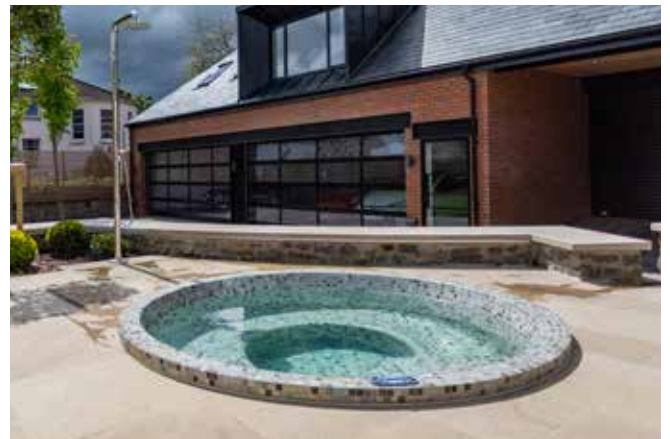
2838 | PRIVATE CLIENT, BRISTOL PROJECT | OUTDOOR POOL & TILED SPA
