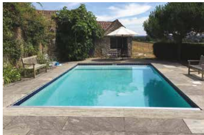
2670 | PRIVATE CLIENT, BATH PROJECT | OUTDOOR POOL RENOVATION
